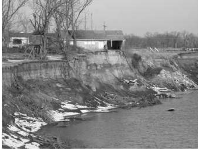
Erosion along Stranger Creek has reached a house along the bank
